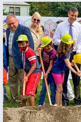
Students help break ground for Pell Elementary School's new building expansion in Newport.
