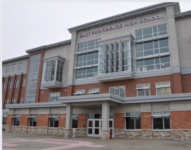
The brand new state-of-the-art East Providence High School has 116 science labs and expanded facilities for career and technical education.
